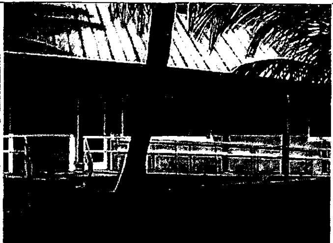
04-04-2014 BLDG. FRONT CENTER VIEW
