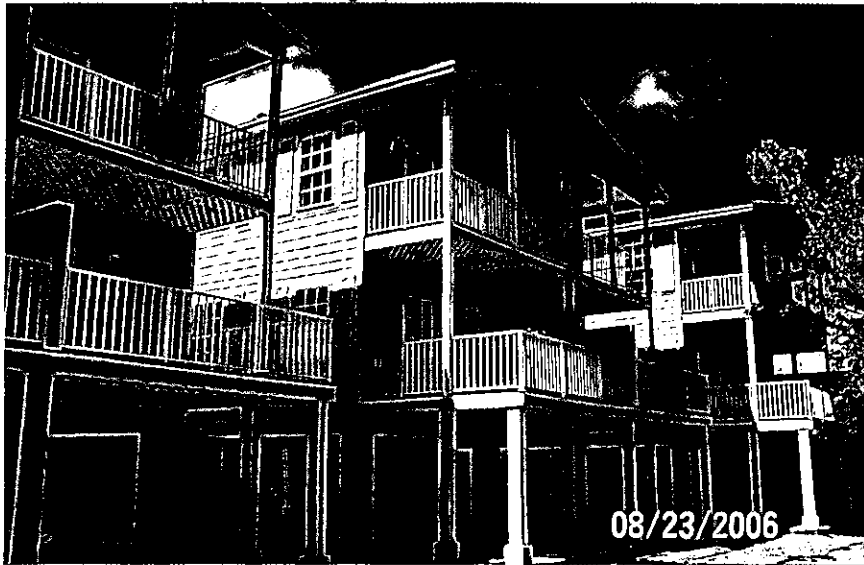
Rear Side View (unit #8 on right)
