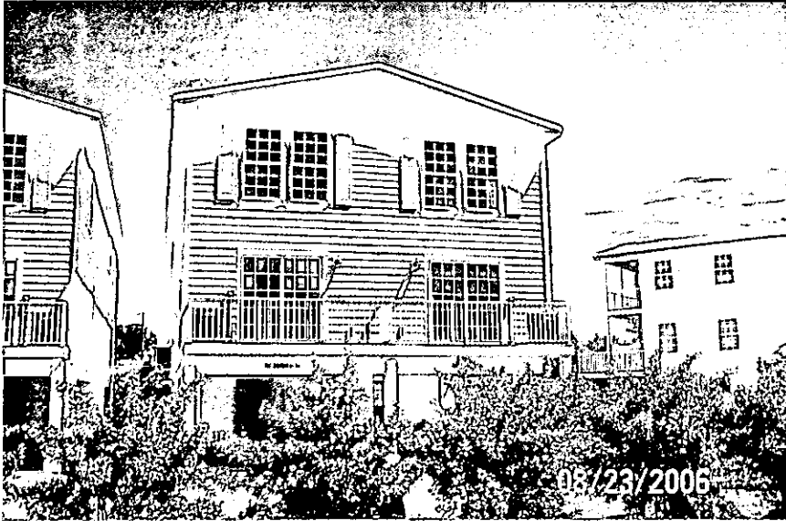
N'ly Road Side View (unit #5 on right)
