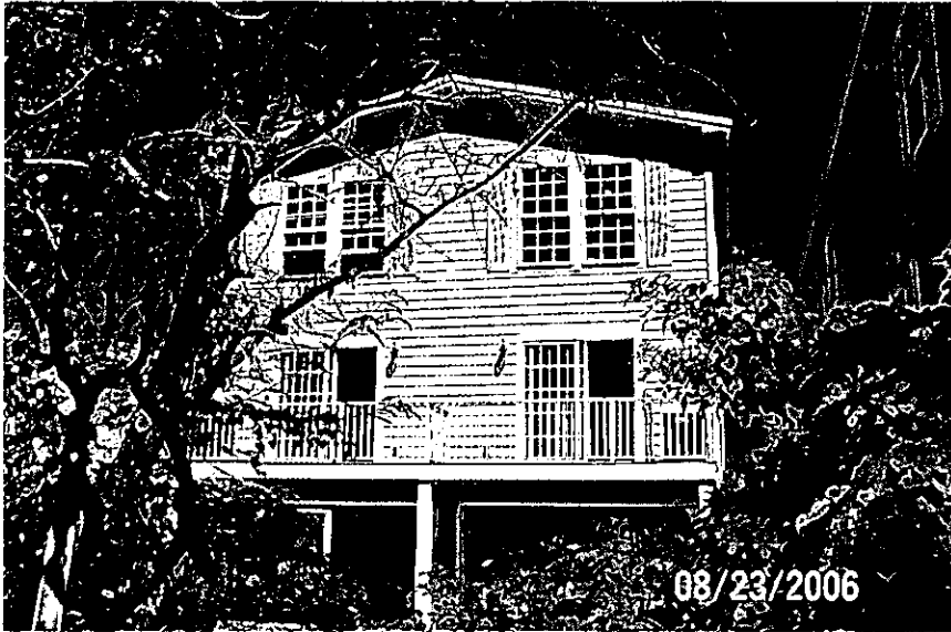
Nw'ly Road Side View (unit #3 on right)
