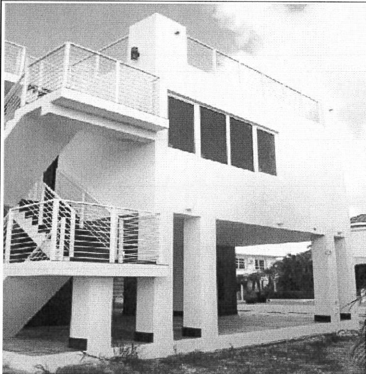
Photo Two Caption LEFT VIEW (06/01/2018)
